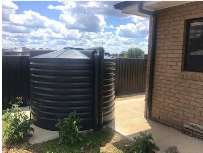
Figure 9: South west corner: Downpipe charged as evidenced by full of water. Rest of the downpipes were not charged with water. Ground near tank noted to be damp.
