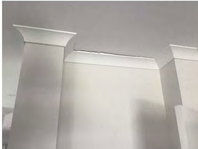
Figure 18: Hall ceiling lifted off linen room wall by an estimated 10mm to cause cornice separation.
