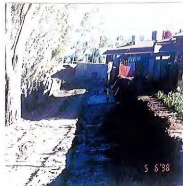
Photograph 21 Dentist Surgery/Courthouse Retaining Wall Construction
