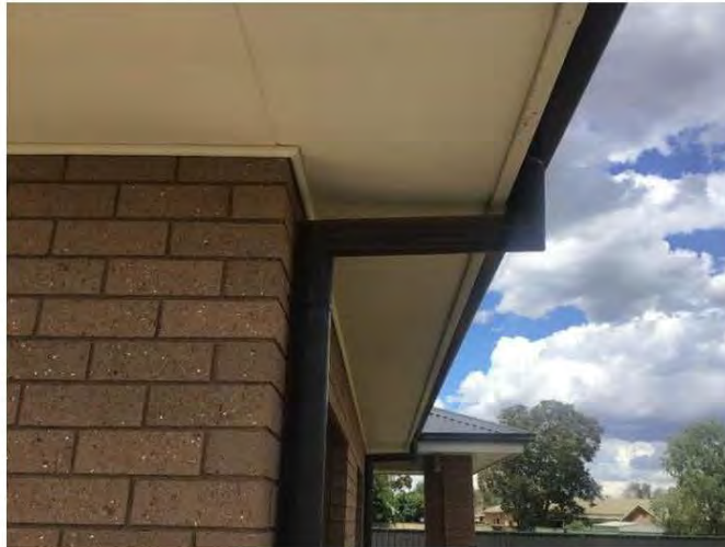
Figure 11: South west corner: Gap to eaves quad 7 to 8mm wide.
