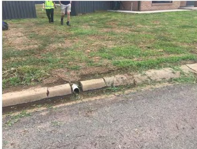
Figure 6: North east corner - Front downpipe discharge pipe to kerb.
