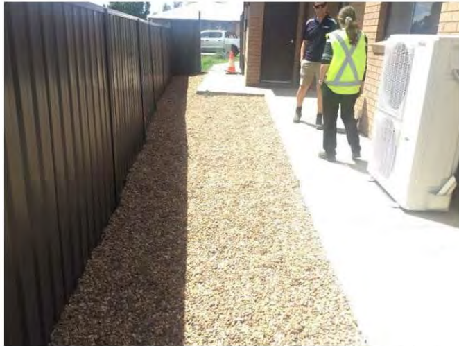
Figure 10: West side gravel with adequate fall away from building.
