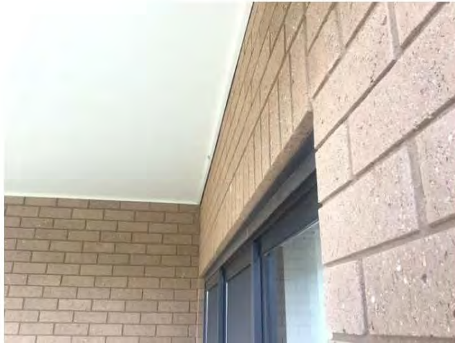
Figure 8: Rear patio at south east corner: Soffit quad gap 10mm to brickwork.
