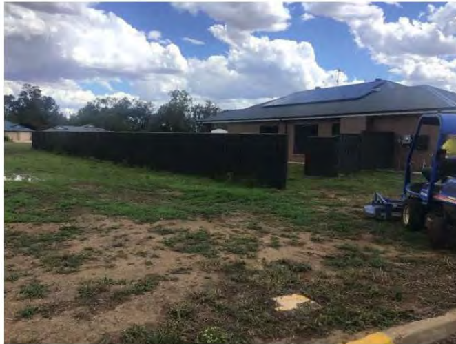
Figure 2: East side neighbouring block with water ponding.
