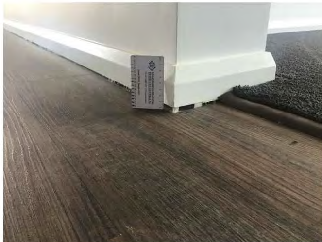
Figure 19: Hall near living room: Wall separated from floor by 10mm.
