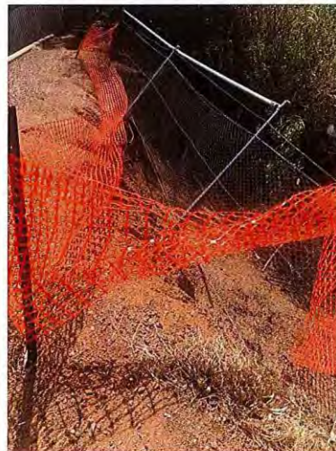
Photograph 5 Dentist Surgery/Courthouse Slippage
