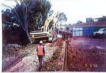
Photograph 18 Dentist Surgery/Courthouse Retaining Wall Construction
