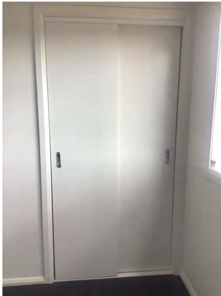
Figure 24: Bedroom No. 4 (west side): Built in wardrobe sliding door gap 5mm.
