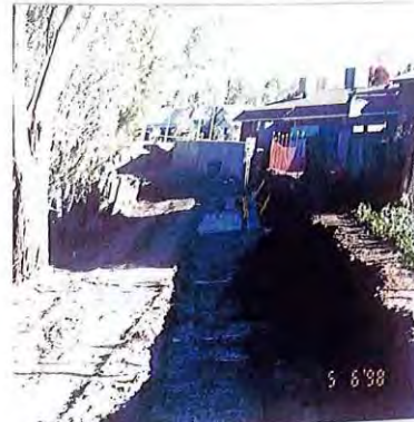
Photograph 19 Dentist Surgery/Courthouse Retaining Wall Construction
