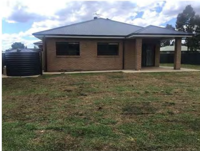
Figure 4: South or rear side. Turf placed, good fall away from building. Sewer boundary trap at rear.
