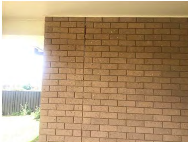
Figure 7: Rear Patio at south east corner: Brickwork articulation joint opened up 10mm at the top.
