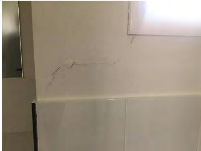
Figure 16: Ensuite: 1.4mm wide crack to east side window.
