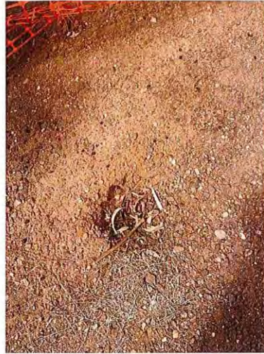
Photograph 11 Dentist Surgery/Courthouse piping
