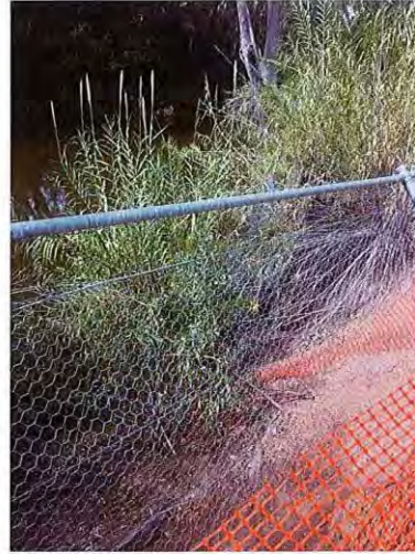
Photograph 7 Dentist Surgery/Courthouse Slippage
