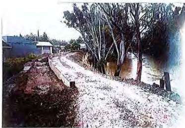
Photograph 20 Dentist Surgery/Courthouse Retaining Wall
