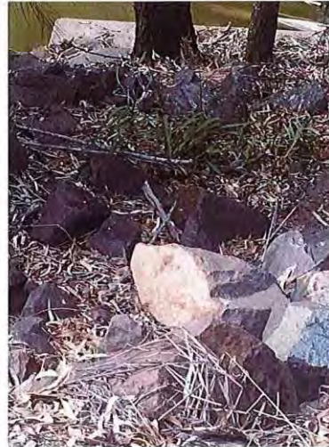
Photograph 15 Lions Park Rock Protection and Sheet Pile Cap Townside
