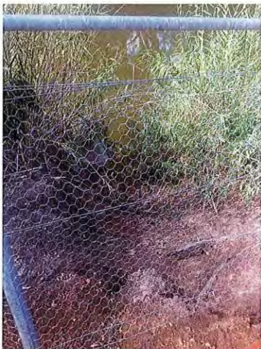
Photograph 8 Dentist Surgery/Courthouse Slippage
