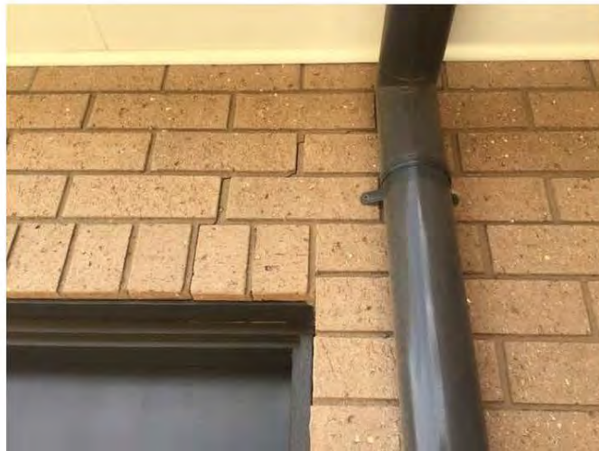
Figure 12: West side - Rear Garage personnel door with brick crack 1mm wide.
