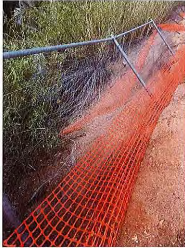
Photograph 6 Dentist Surgery/Courthouse Slippage
