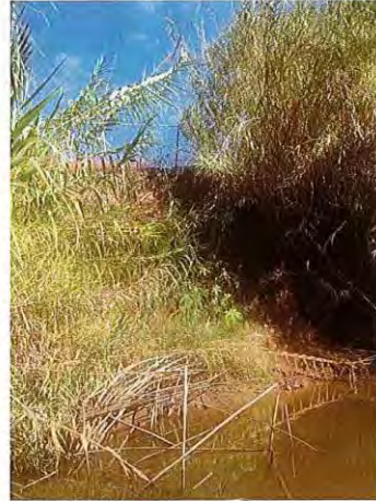
Photograph 3 Dentist Surgery/Courthouse Slippage
