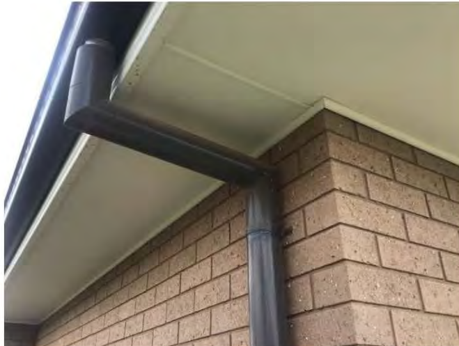
Figure 5: North East Corner downpipe bracket moved upwards, covered with more recent paint.
