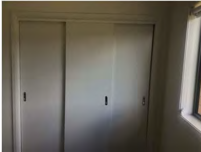
Figure 22: Bedroom No. 2 (rear middle): Built in wardrobe sliding door with 10mm gap at top near rear wall.
