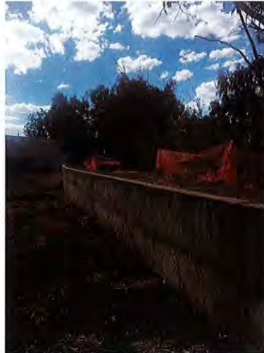
Photograph 13 Dentist Surgery/Courthouse Retaining Wall
