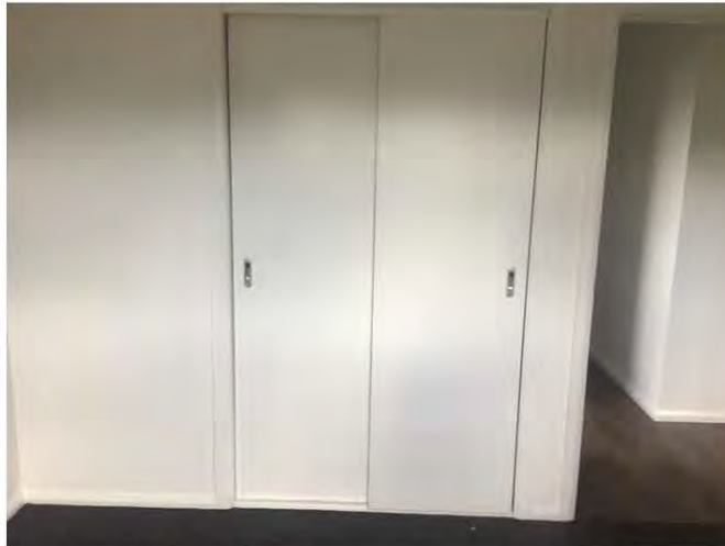
Figure 23: Bedroom No. 3 (South west corner): Built in wardrobe sliding door gap 6mm. Door sticks at bottom.
