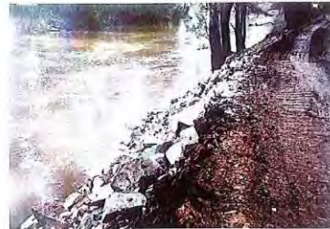
Photograph 23 Typical Levee Construction Riverside
