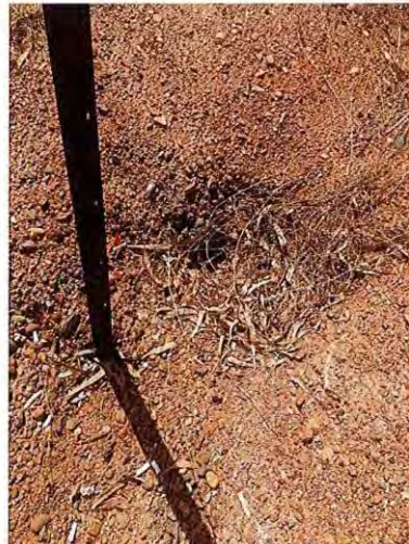
Photograph 9 Dentist Surgery/Courthouse piping
