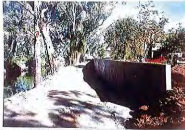
Photograph 22 Typical Retaining Wall Construction
