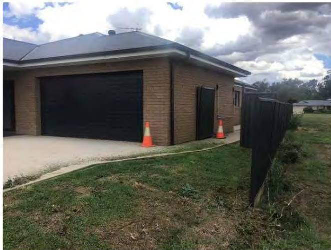
Figure 3: West side gravel outside external concrete slab and steeper fall to boundary.
