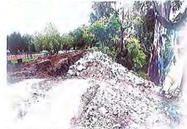
Photograph 24 Typical Rock Protection of Levee Riverside
