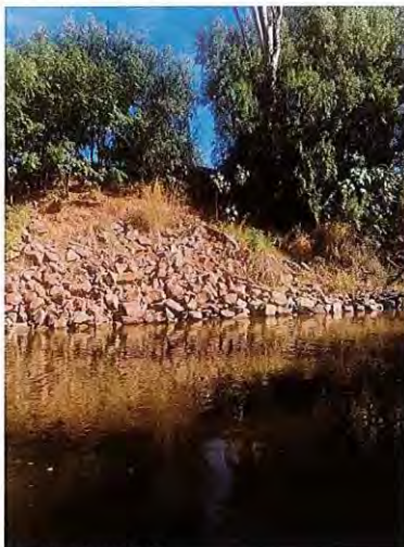
Photograph 25 Typical Rock Protection Riverside
