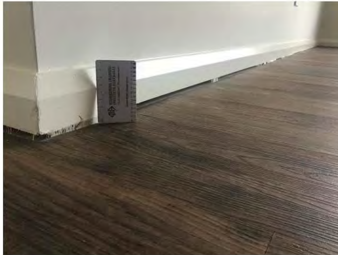
Figure 20: Dining room: Living room wall separated from floor by up to 8mm, zero gap at east end.
