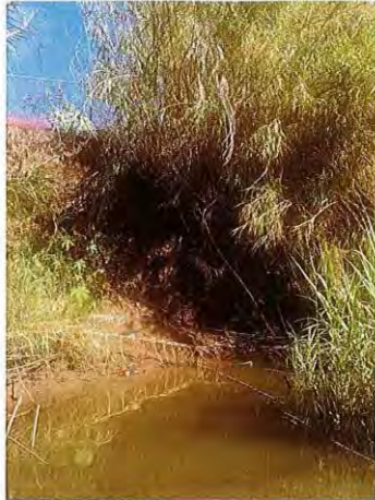
Photograph 2 Dentist Surgery/Courthouse Slippage
